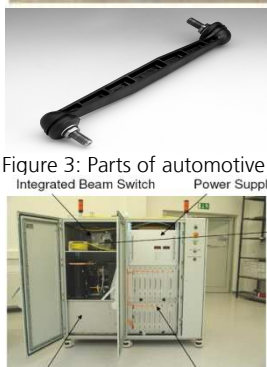
Figure 4: Laser system Integrated Compressor Chiller Modules
